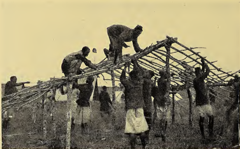
Building a Grass House
